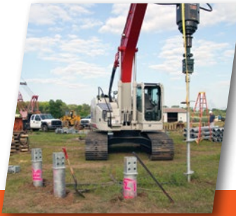
Helical pier installation
