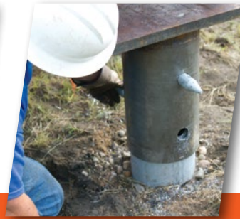
Adapter caps secured on piers
