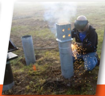
Pier top removal by plasma torch
