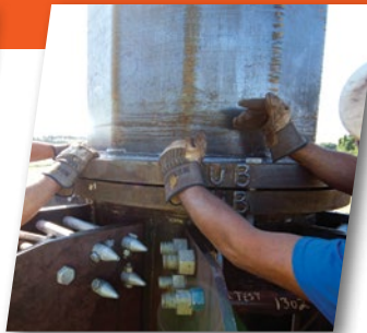
Pole quickly connected to adapter
